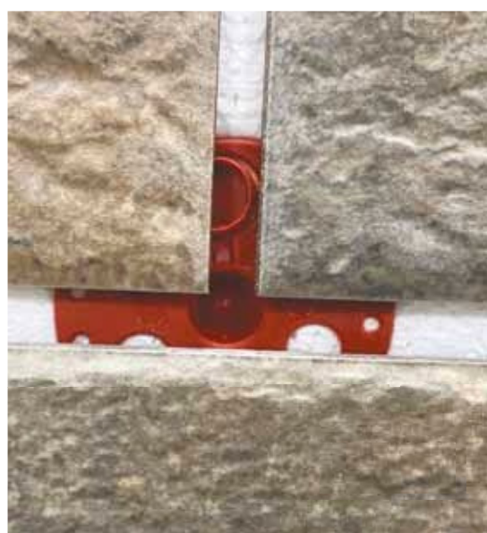
Picture 2. Embedded detail in clinker thermopanel
