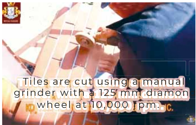
Picture 1. Thermopanel cutting: lines of saw-cutting for external corner formation
